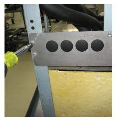
• Remove screws around perimeter on top of the water tank. Remove the temperature probe from top of the tank and set aside.
