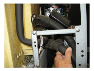
Open cabinet door and disconnect the water line coming into the back of the cabinet at the tee and remove line through the back of cabinet. Disconnect the motor harnesses located in the back of the cabinet. Push the connector through the back of the cabinet.
