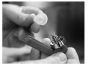
6. Remove the old faucet seat cup from the handle and bonnet assembly and replace the seat cup with a new one. Reinstall the seat cup to the faucet assembly by pressing firmly to ensure a proper connection (should interlock). Reinstall the handle and bonnet nut assembly rotating the nut clockwise to hand tight.
